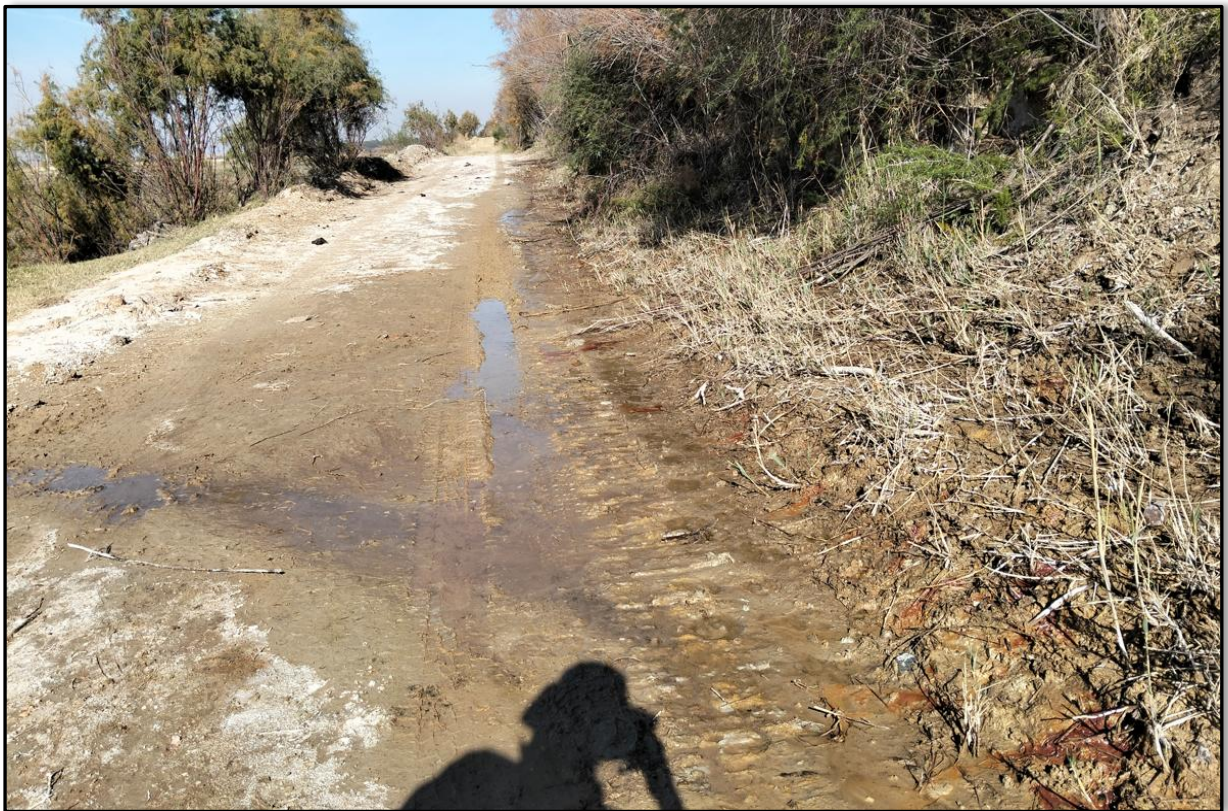
Plate 5. Seepage along the toe of the upper compartment embankment near test pit TP32.
