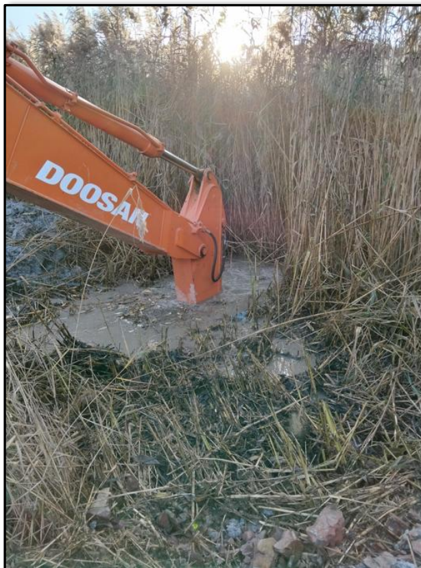
Plate 48. Saturated test pit at TP24.
