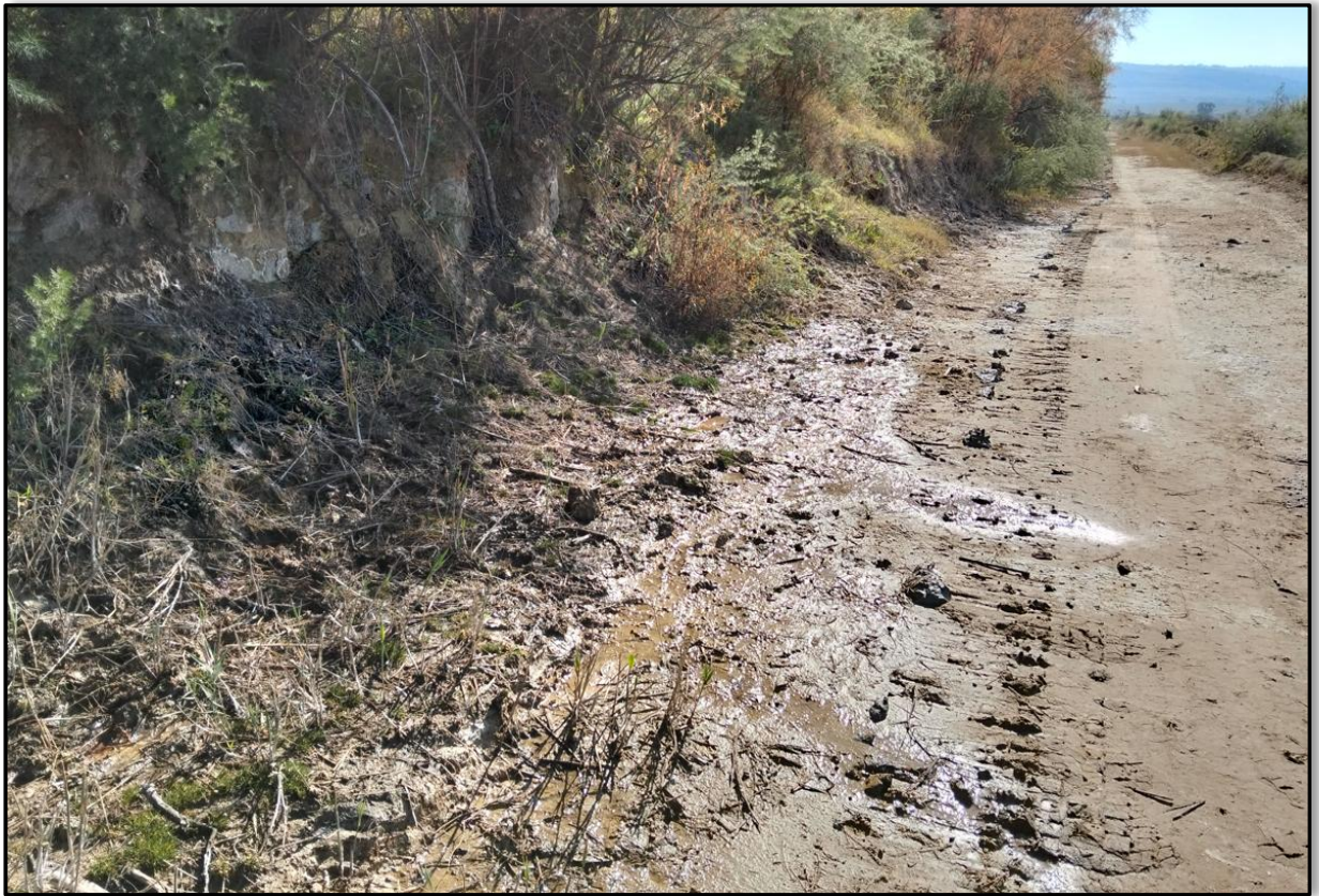
Plate 6. Seepage along the toe of the upper compartment embankment near test pit TP32.
