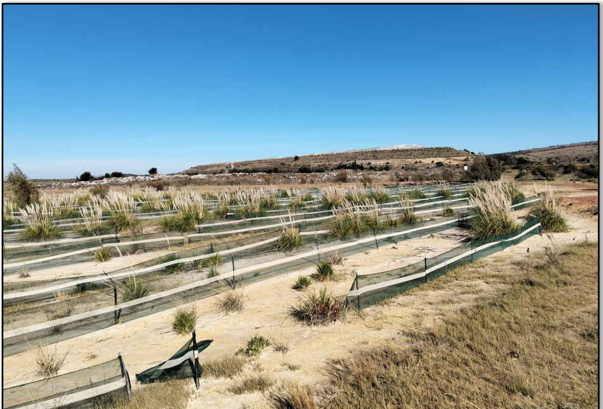
Plate 11. Paddocks at test pit TP12 with erosion control measures.
