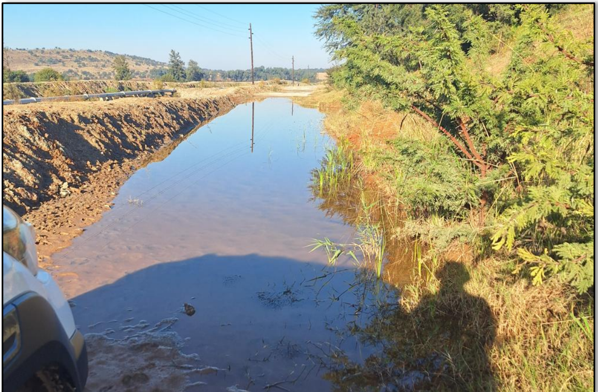
Plate 29. View of abundant seepage below the starter wall at south-eastern embankment.
