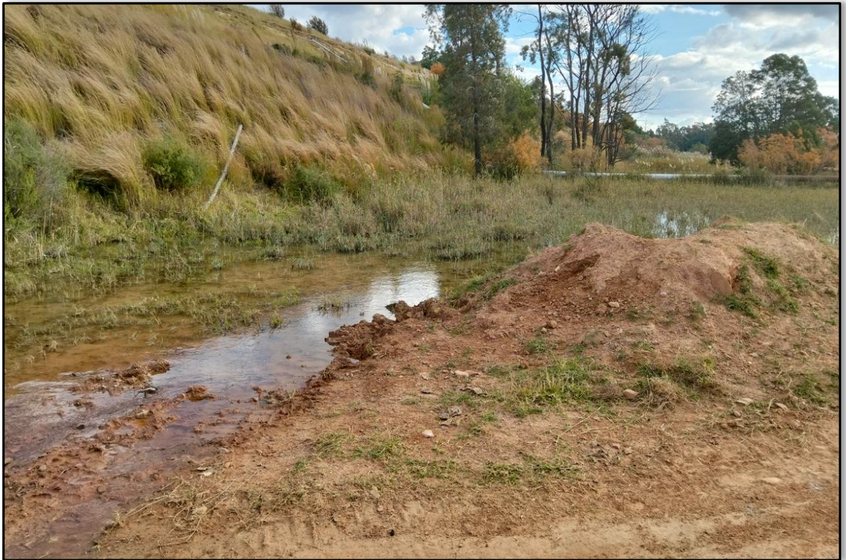
Plate 2. Water seepage at the lower compartment entrance.
